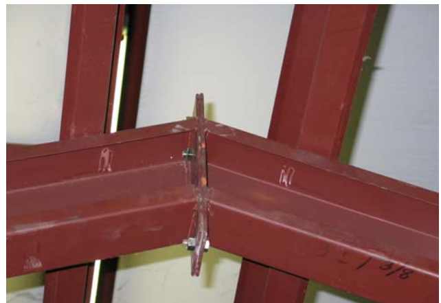
STANDARD SECTION @ RIDGE ENDWALL
