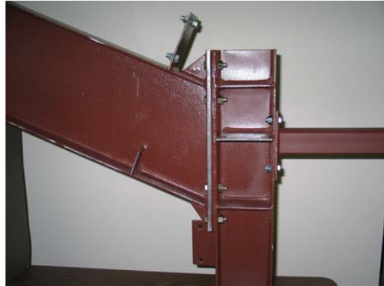
STANDARD EAVE SECTION @ FRAME
